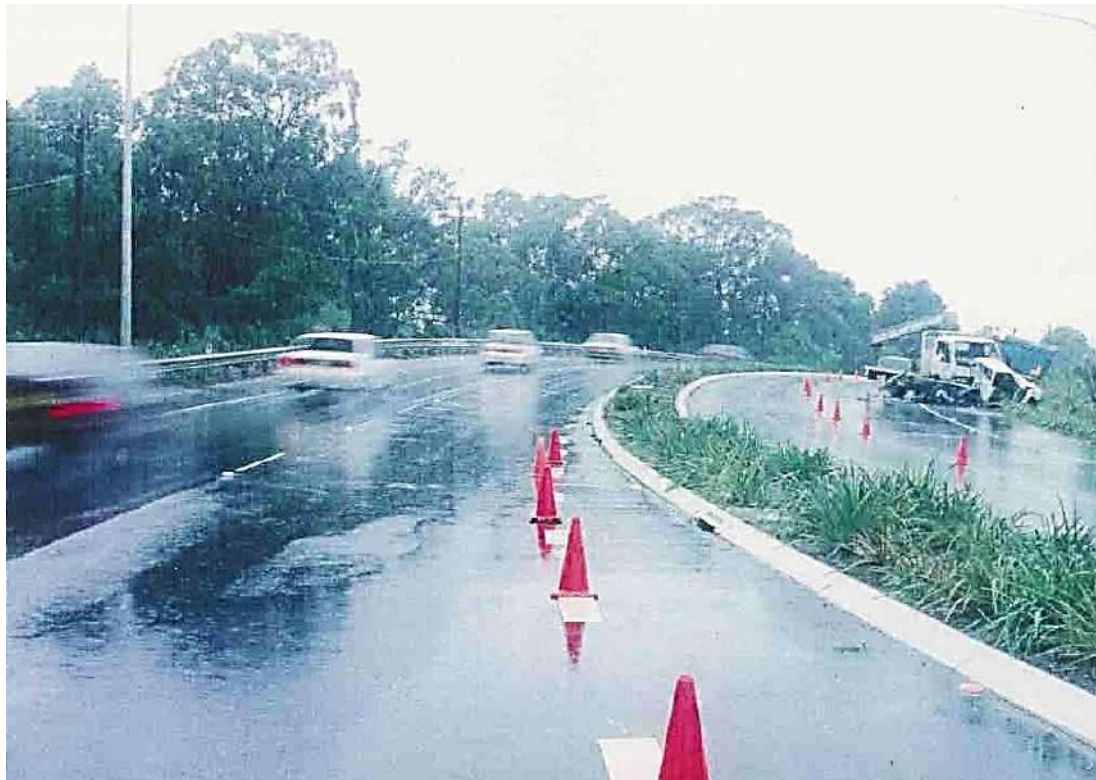
Figure 1a: Water pooling on lanes left of median.
