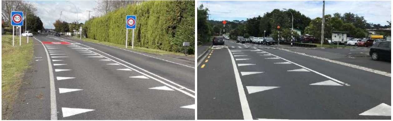
Figure 1. Dragons Teeth at speed thresholds (left) and school pedestrian crossing (right).
