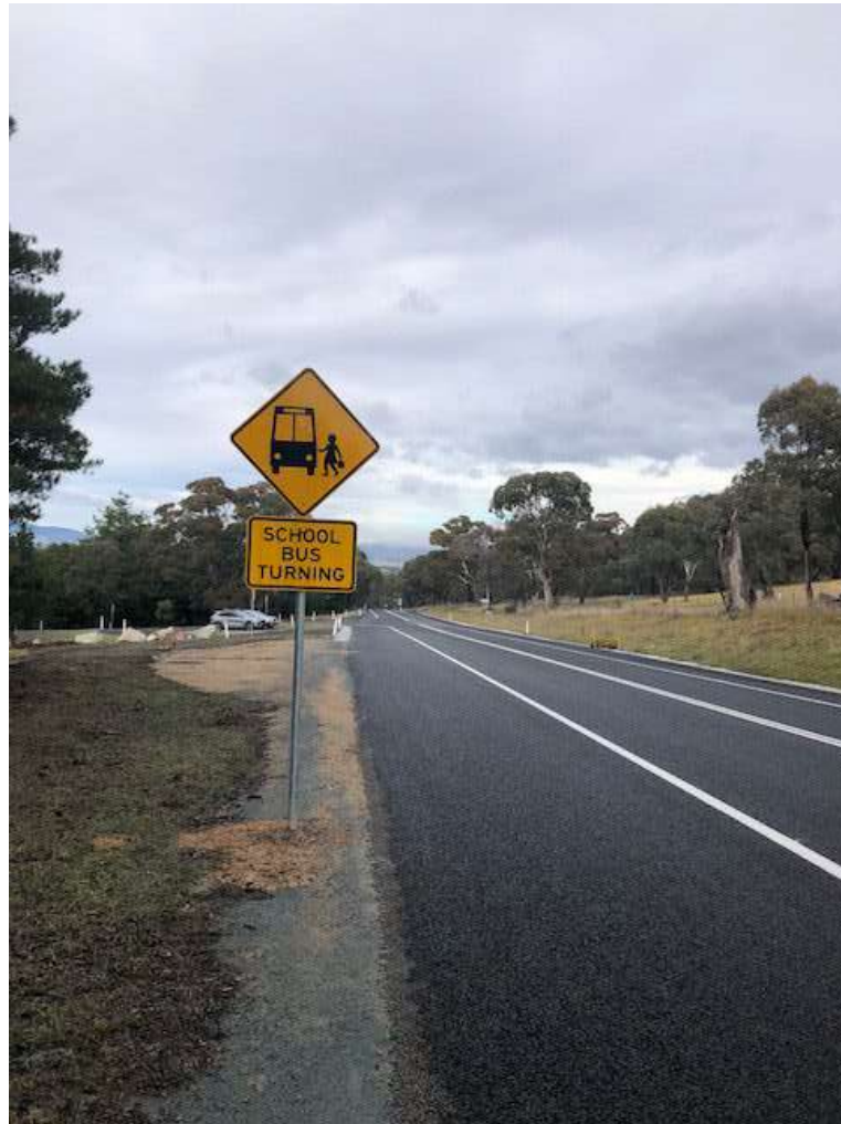
Figure 1. Identified crash risks eliminated for informal bus stops on a high-speed rural road
