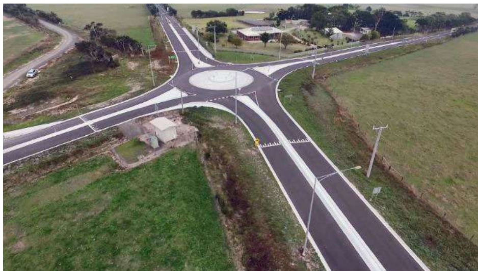
Figure 1. Lance Creek compact roundabout. Note the raised safety platforms on approach and the elongated splitter islands.
