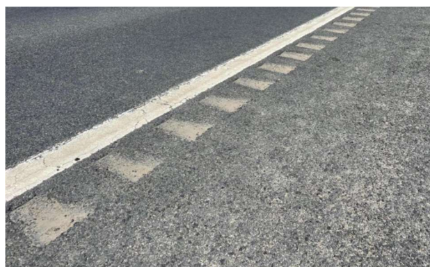
Figure 4: Traditional Milled ATLM treatment
