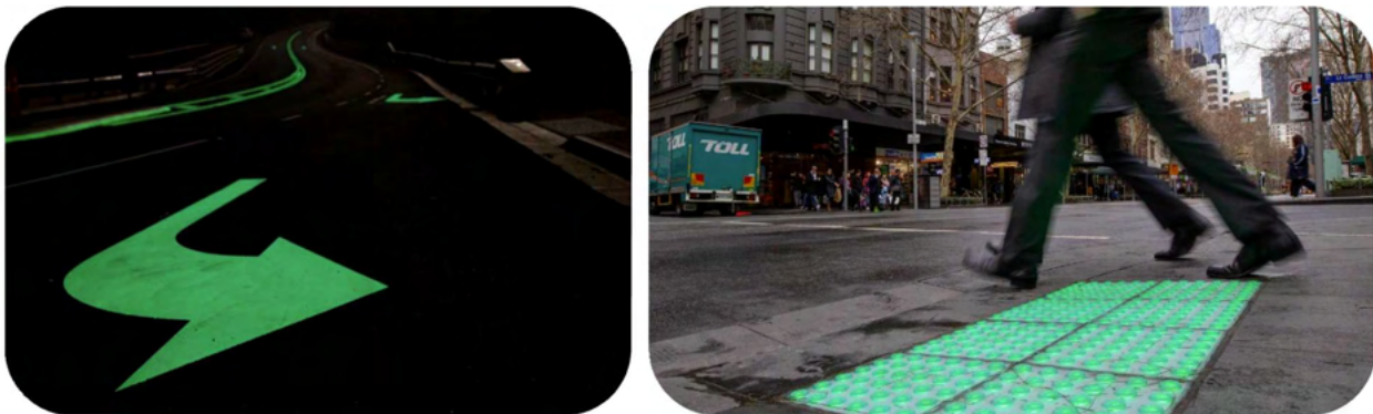
Figure 1. Example of PL linemarking (left image) and pedestrian TGSI (right image)
