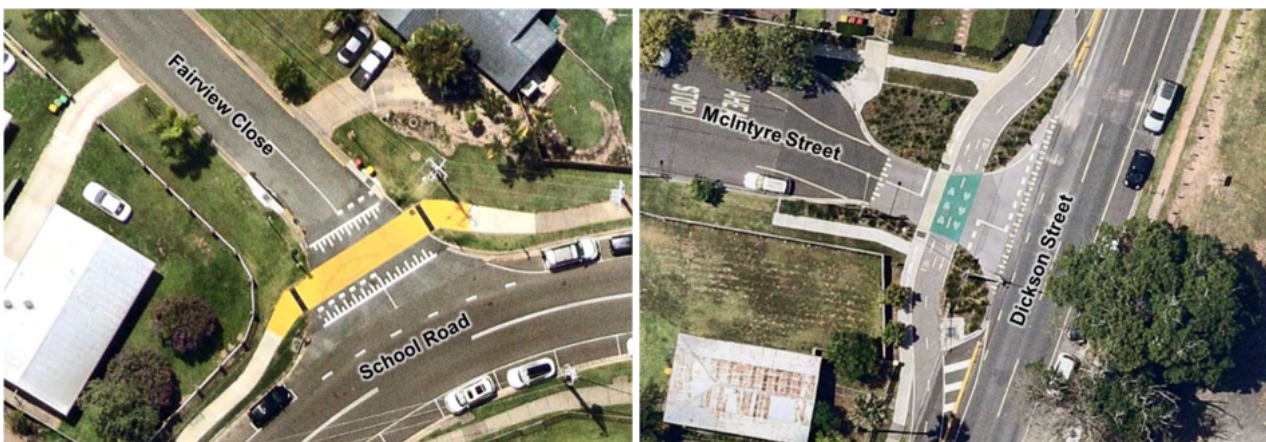
Figure 1. Fairview Close and School Road Priority Crossing, Bli Bli (Left) and McIntyre Street and Dickson Street, Wooloowin (Right)
